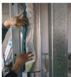
Wrap each segment with an overlap
